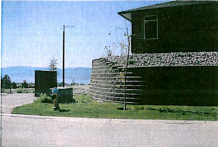
Artificial grading to improve views to the Lake creates a visual impact from the street
