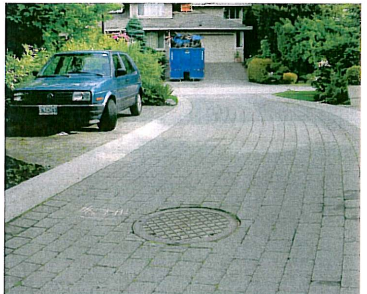
Narrow pervious road surface with parking bays
