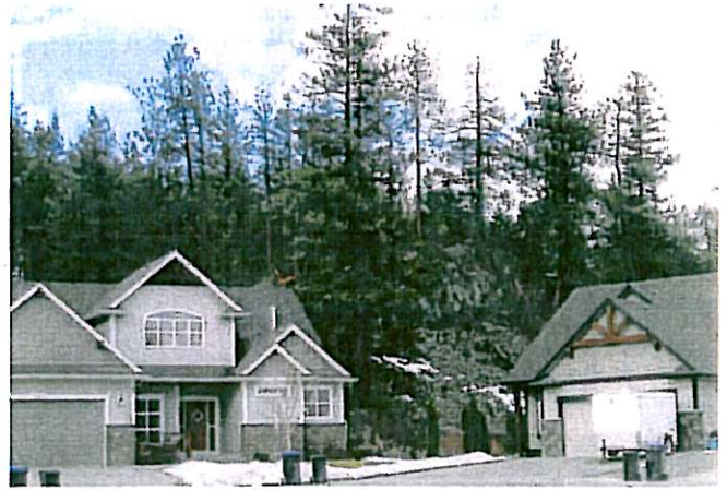
Natural slope retained between houses
