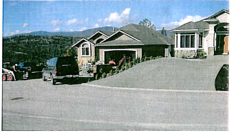
Driveway slope does not respect natural terrain
