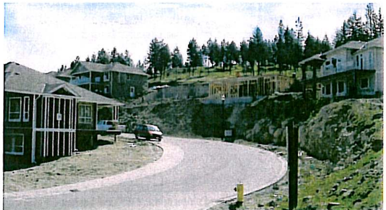
Stringent road standards may contribute to instability concerns
