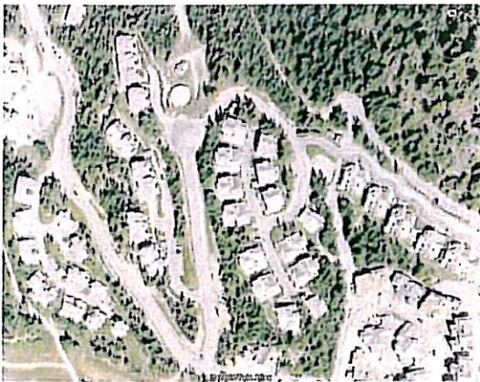
Alternate road design accommodates difficult terrain
