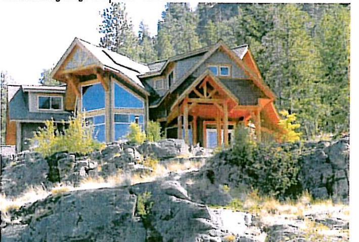
Attractive building articulation
