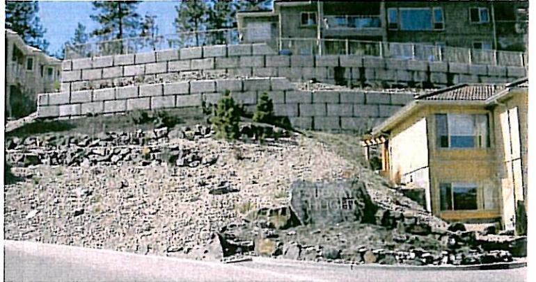
Unattractive, visually dominant retaining wall
