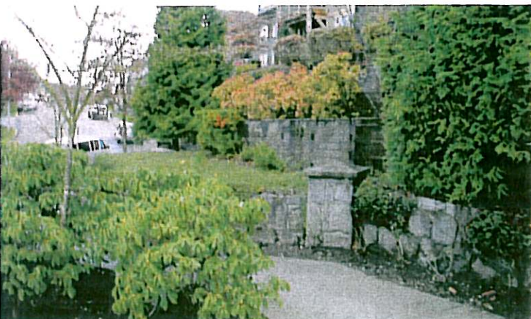
Large retaining structure effectively screened with landscaping
