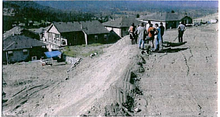
Potential slope instability
