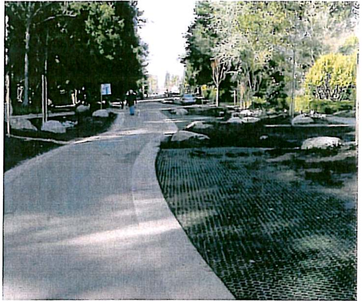
Automobiles tolerated with narrow pavement width and parking bays
